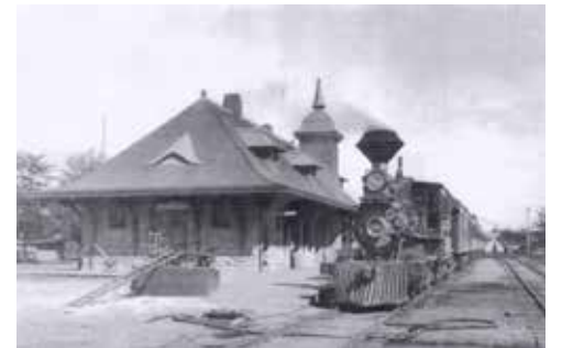
Oregon Short Line Railroad Station, Boise.
